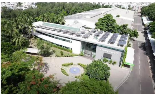
Grundfos Pump at Chennai.
